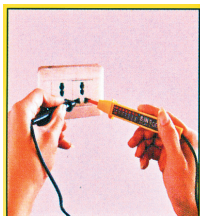
TEST AC VOLTAGE
